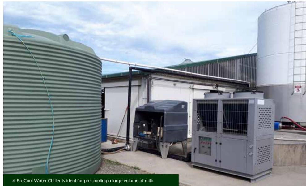
A ProCool Water Chiller is ideal for pre-cooling a large volume of milk.
